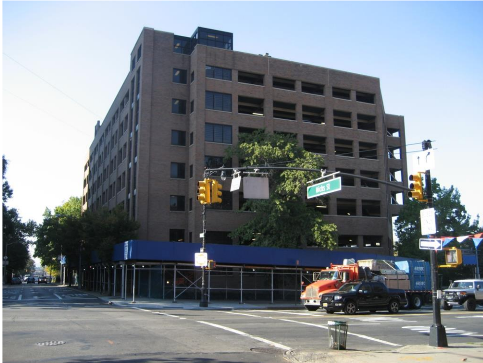
Parking Garage Facing South from Atlantic Avenue
