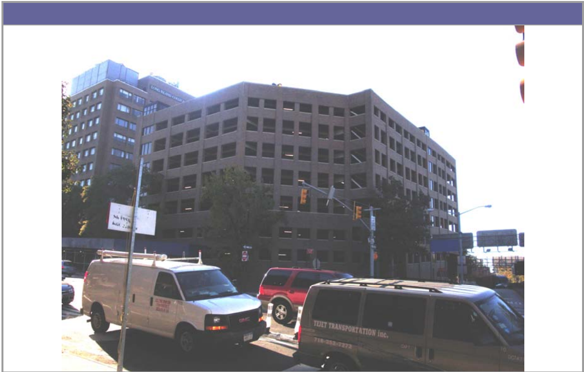
View of subject property looking southeast across Atlantic Avenue
