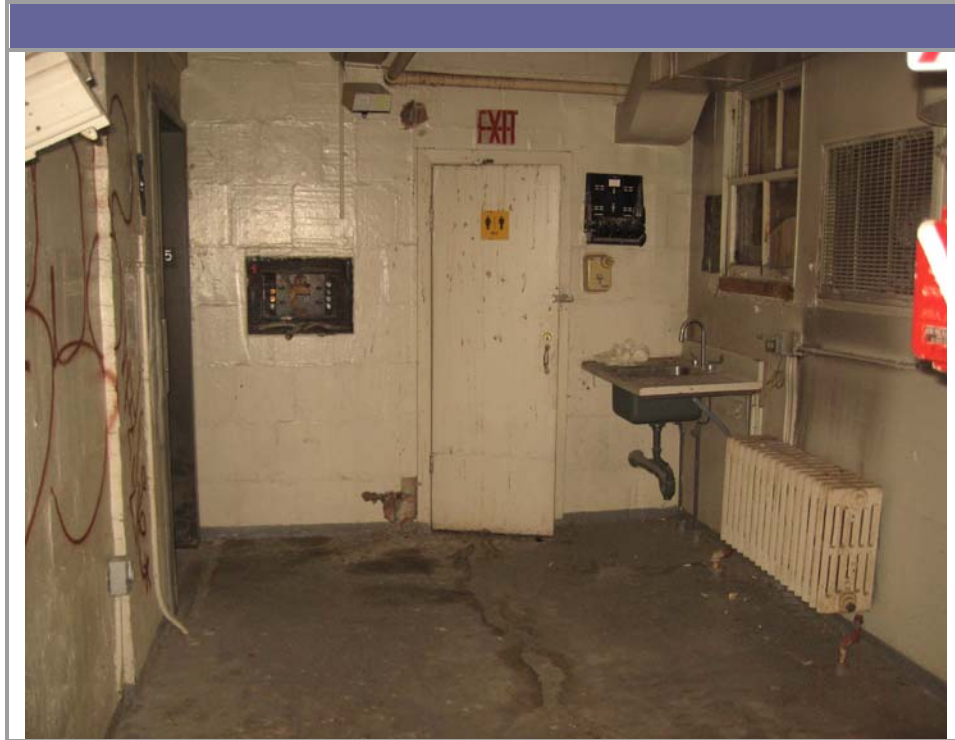
View of a former treatment room
