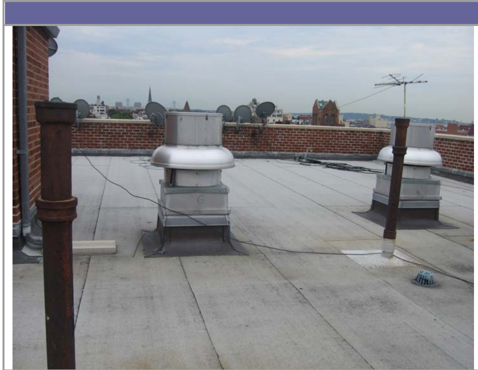
View of the roof
