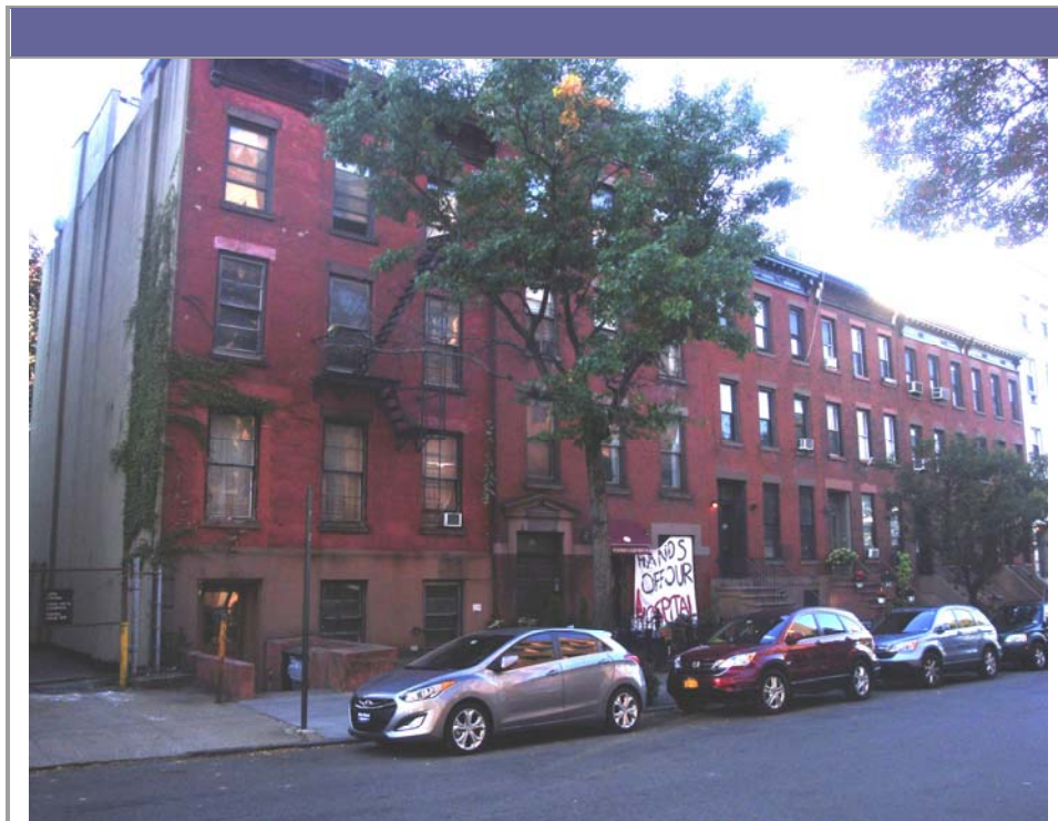
View of the subject facing southwest across Amity Street
