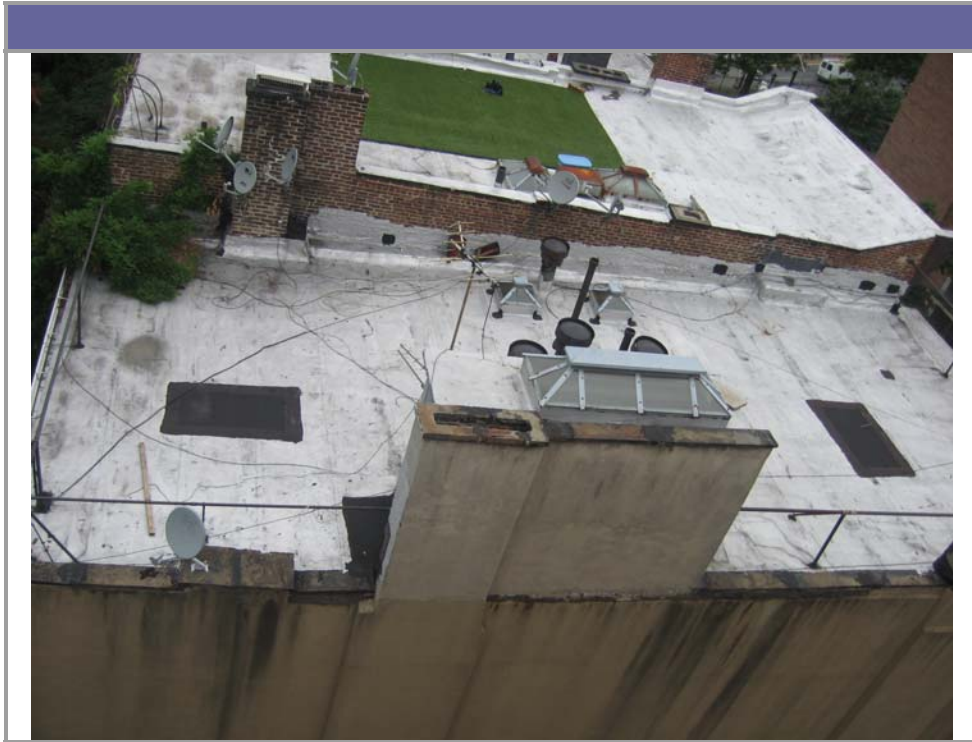
View of the roof
