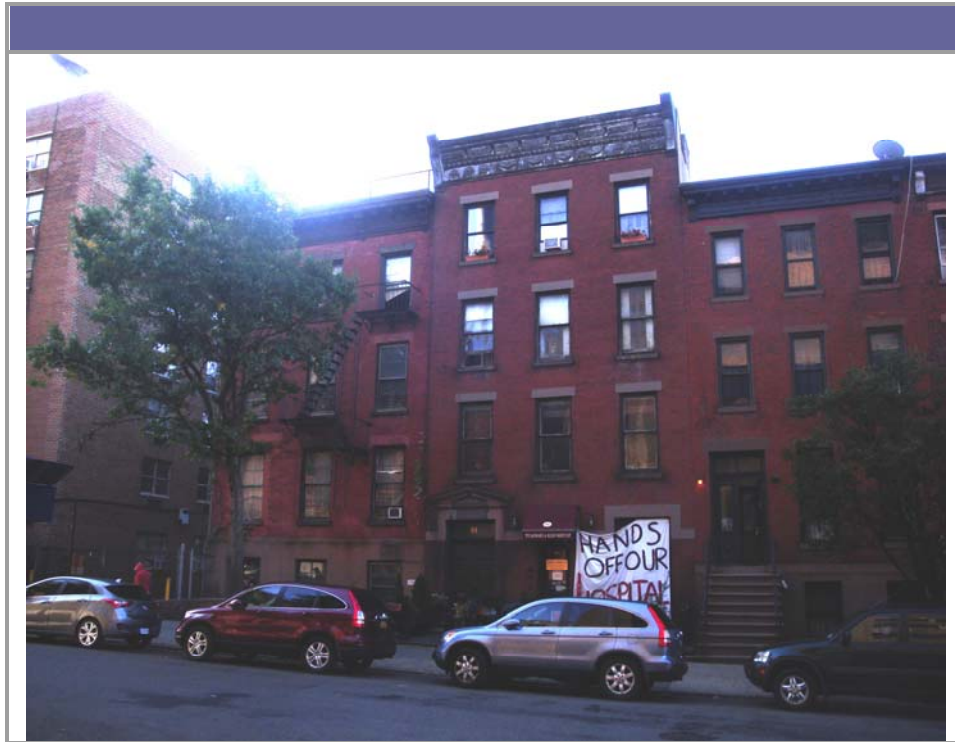
View of the subject facing southeast across Amity Street
