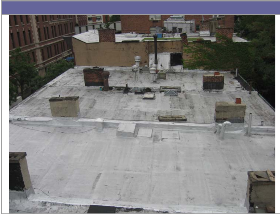
View of the roof
