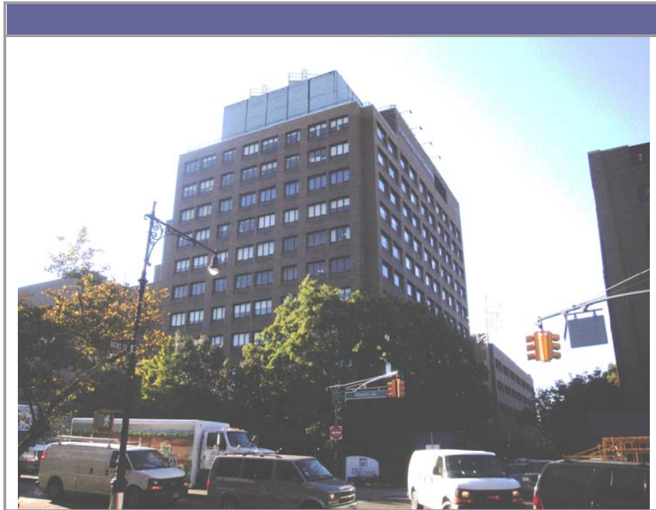
View of the subject facing southeast across Atlantic Avenue and Hicks Street
