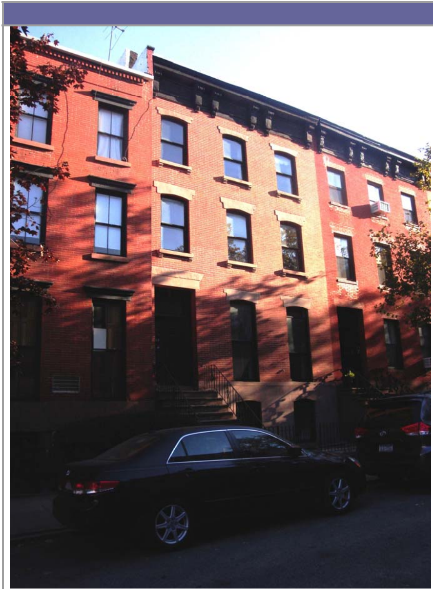
View of the subject facing northeast across Congress Street
