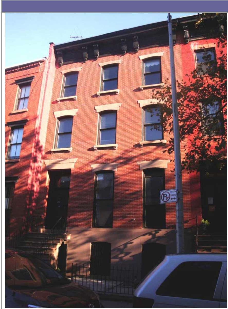
View of the subject facing northwest across Congress Street
