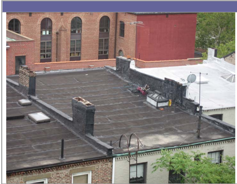
View of the roof
