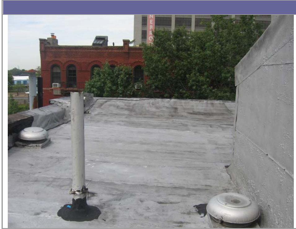
View of the roof
