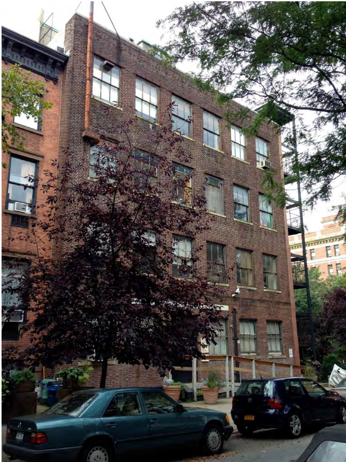
112 Pacific Street as viewed from Pacific Street
