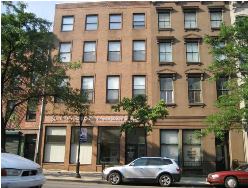
130-134 Atlantic Avenue – Front View
