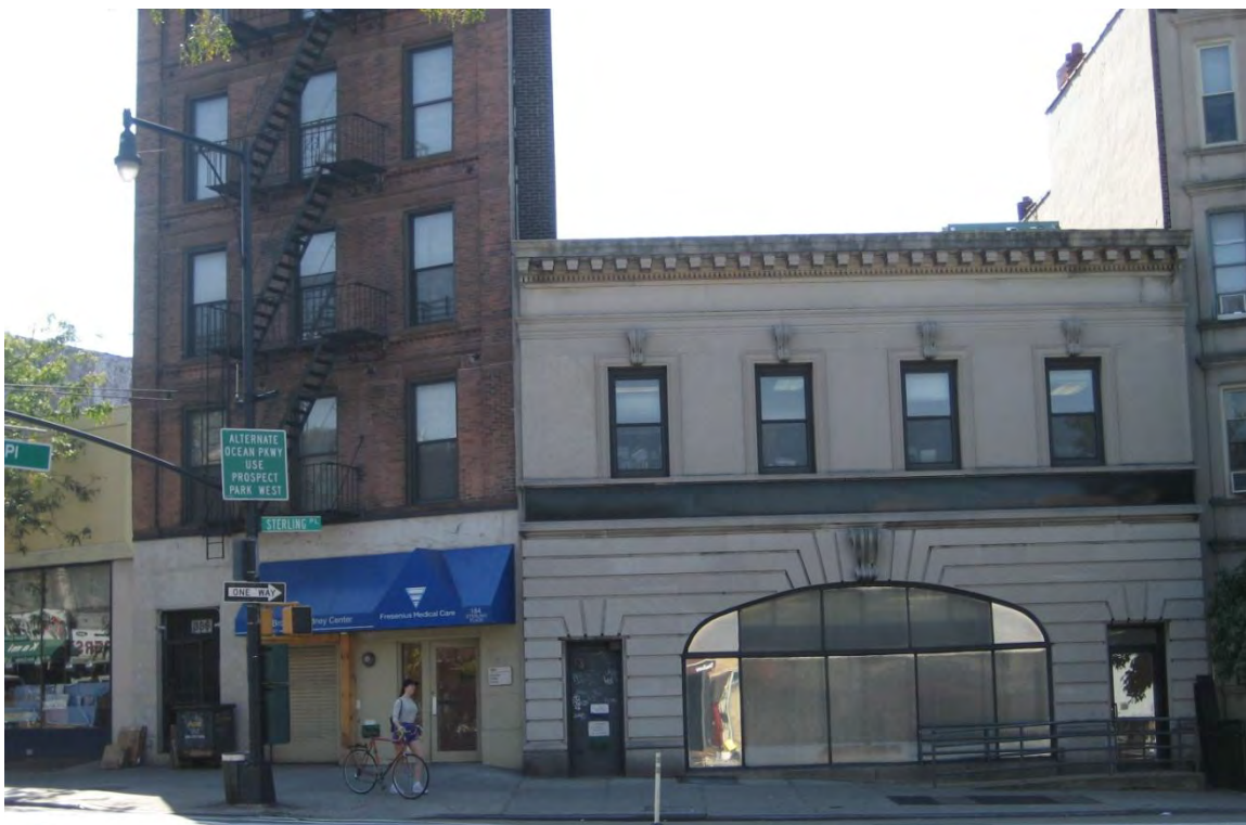
336 Flatbush Avenue and 184 Sterling Place
