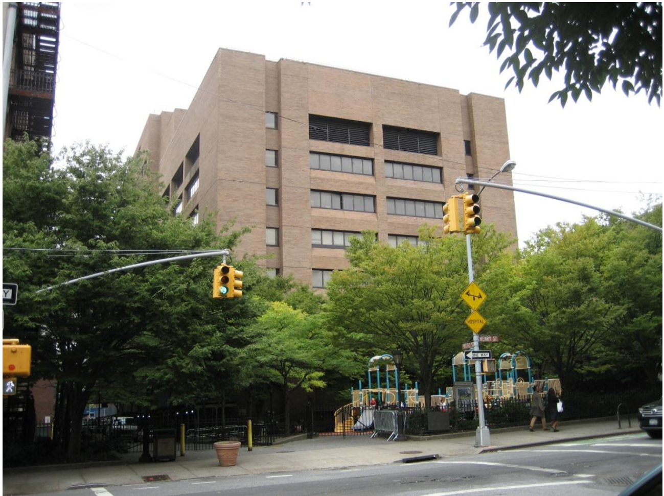
Othmer Building – 91-95 Pacific Street
