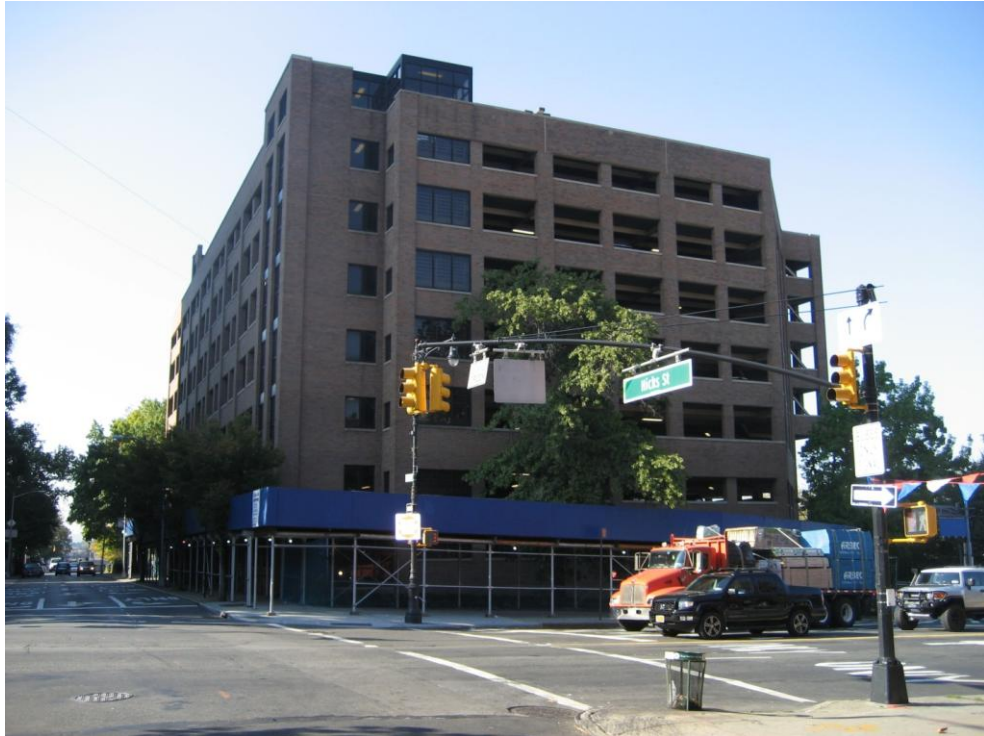
Parking Garage Facing South from Atlantic Avenue
