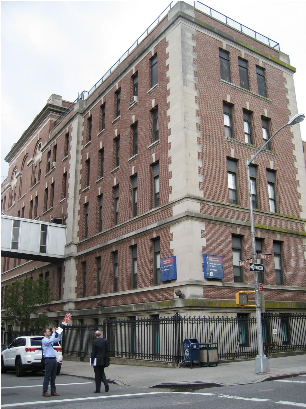
340 Henry Street Facing North from the Northwest Corner of Amity Street
